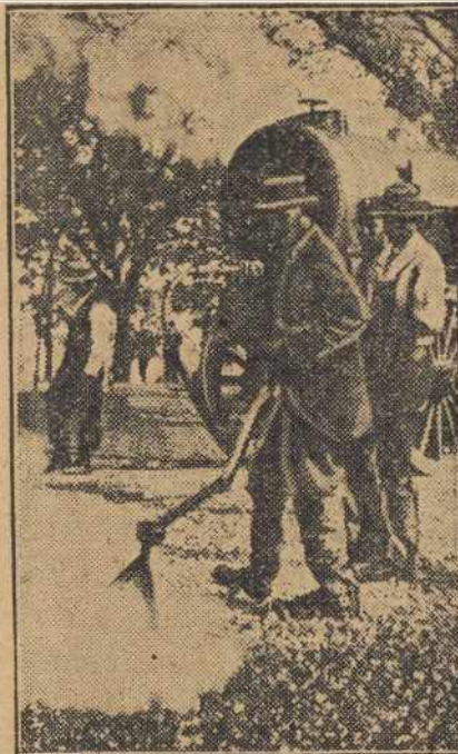
Building a Better Road.
