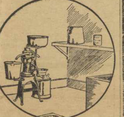
Separator in Clean Room.
