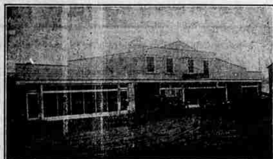
ALBANY GARAGE Now in charge of Hammel and McIntosh
