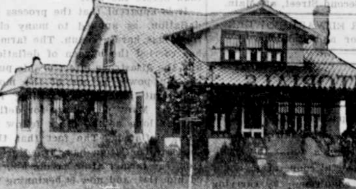
This bungalow is a combination of stucco with a tile roof. The contrast between the stucco and the tile roof is very attractive.
