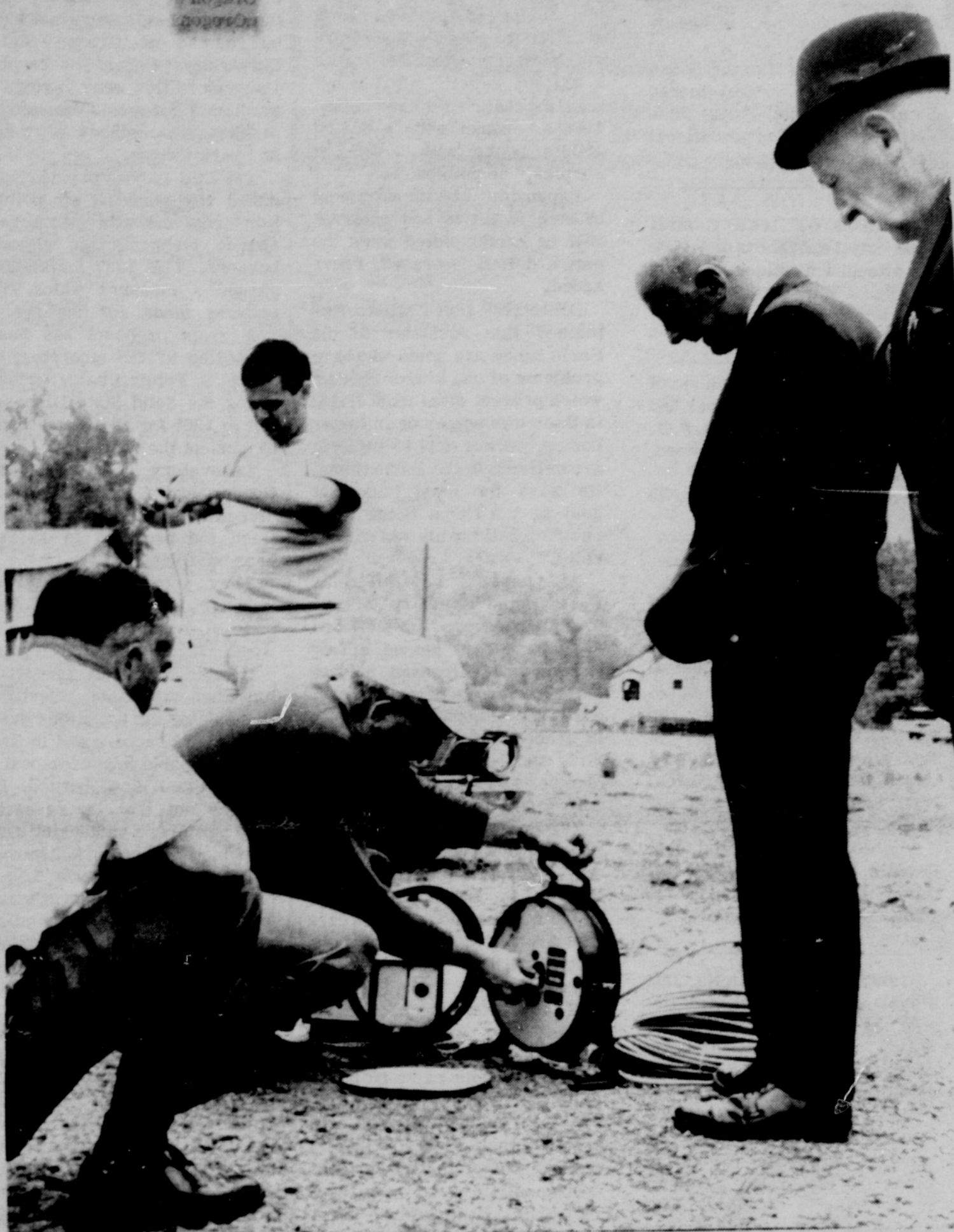
PORTLAND GENERAL ELECTRIC COMPANY people were interested spectators when R. T. Jaske, Battelle Northwest scientist, calibrated thermograph being installed as first step in $92,000 environmental study under way in the Columbia river. PGE is financing the study in preparation for construction of one-million-kilowatt nuclear generating station between St. Helens and Rainier.
