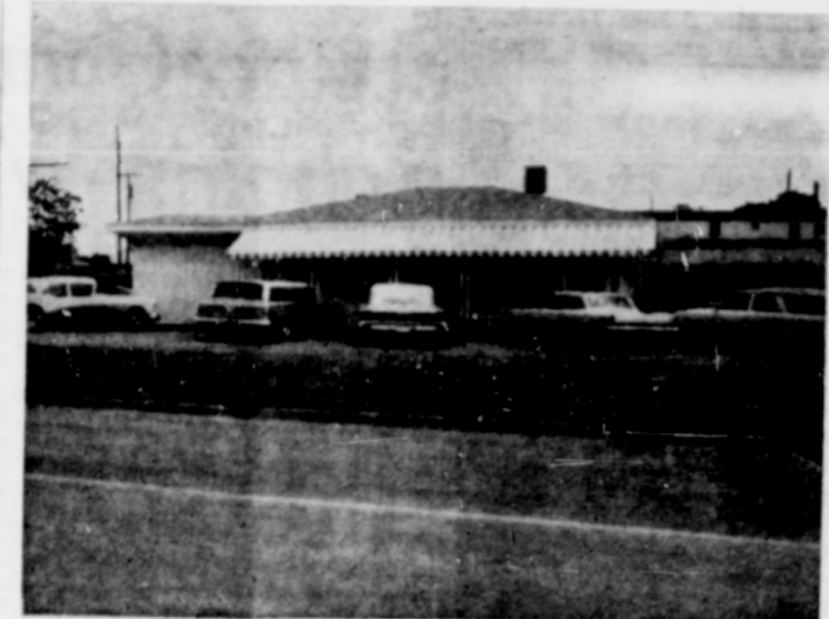
ONE OF WASCO'S big improvements recently was the installation of a California type awning at the Town and Country Grill operated by Mrs. Helen Rich.
