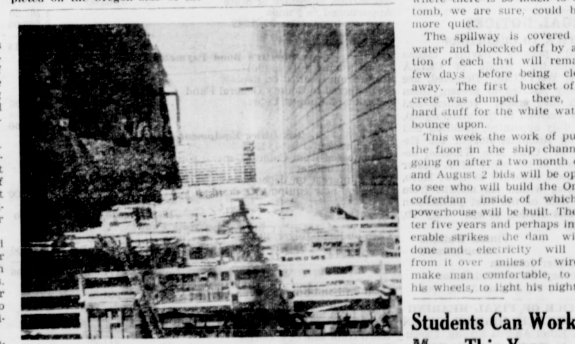
The ship channel is 105 feet deep, 86 feet wide and 675 feet long, the standard for Columbia river dams. The forms are for the floor of the locks on which work can start again with the ending of the steel strike.
