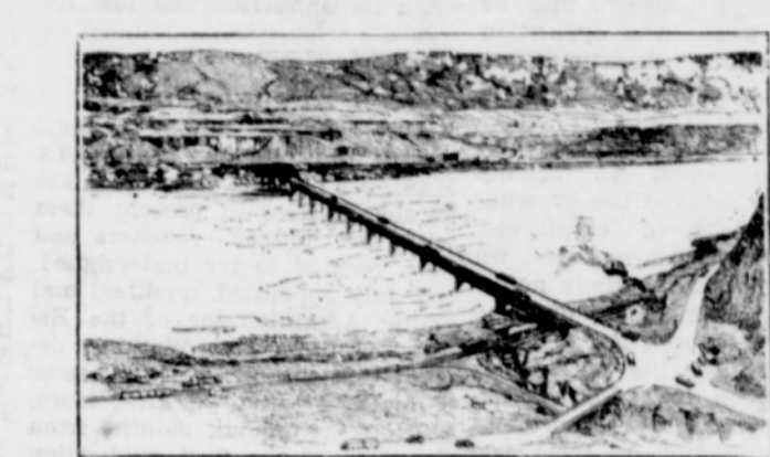
A well known highway engineer drew the plans for the first projected bridge across the Columbia at Maryhill or Biggs Rapids as pictured above. The big depression killed the first
