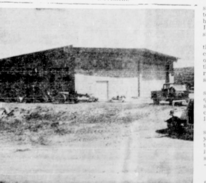
This is the new machine shop Irzyk. It has a five ton hoist, full concrete floors, all the lighting to permit a worker to see anywhere.
