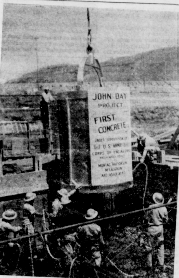
The first concrete ran slowly out of the opening gates of the bucket and the workmen waited until it dropped. The air hose, being held by the man on the top, connects with the gates. Pressing the button to drop the concrete was Mrs. Paul Giannola, wife of the batch plant operator, for four ton buckets.
