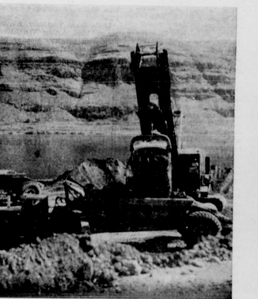
This is the six yard shovel of the 34 yard trucks. Cost of equipment in this picture is over $400,000.
