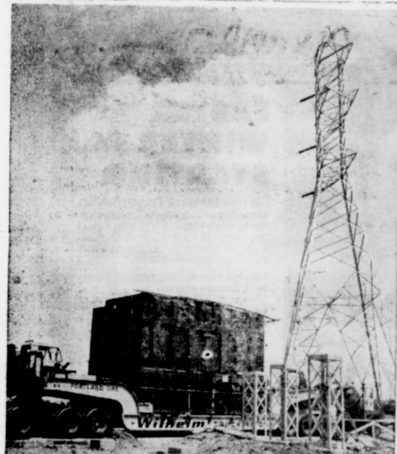
Massive bulk of the largest 000-volt installation in Oregon transformer of its type in the achieve dramatic emphasis for Northwest and the soaring steel PP&L's record system expansion. Terminal tower for Pacific Power Lines will bring new power supply into Oregon system.
