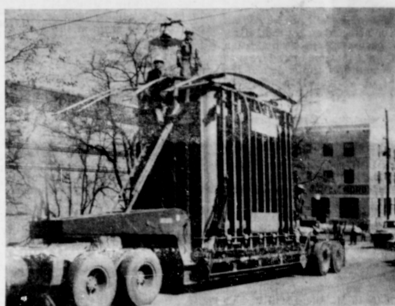
A 400 horsepower tractor and transformer to its destination. 24 tires were used to tow the Here it is on First street.
