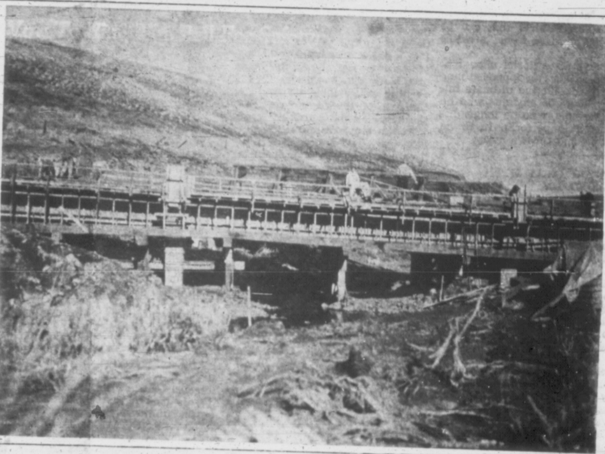
Workmen are tamping in the last section of concrete topping on the bridge across Grass Valley canyon taking concrete from a truck just out of the picture on the left. The state inspector, in yellow shirt, and workmen are raking topping to make it rough. Bridge was raised about three feet from first plans in order to give more clearance for water. Bridge is longer than the one it will replace.
