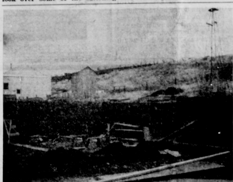
A new and modern house is rising to replace the old and demonstrates an intent to remain on the farm and make it better and more productive.
