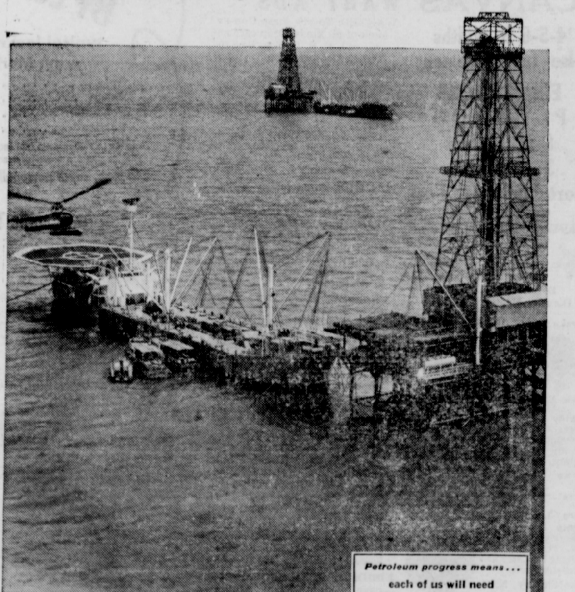
Our search for oil has led to drilling offshore wells like this one (in the Gulf of Mexico) costing nearly 6 times more than land wells.
