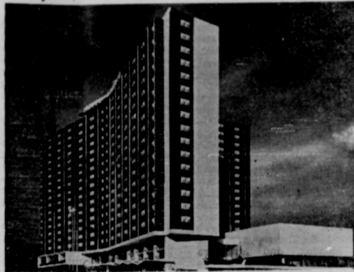
This is a scale model of the 1,001-room Hotel Statler in Dallas, Texas, where each guest room will have television-radio. The hotel will be completely air-conditioned. New type bathrooms will have a dressing room atmosphere. The main banquet area will seat 2,000 in one group. "Flat-slab cantilever" construction to be used for the first time.
