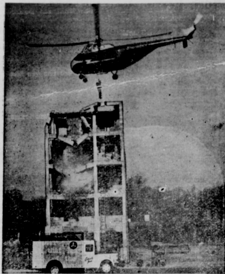
CIVIL DEFENSE ROLE . . . A helicopter is demonstrating one of the ways in which it can be used in civil defense rescue work. The 'copter is lowering a rescue worker to the upper floor of a "wrecked" building in Olney, Ind., to aid people supposedly trapped there. The building is one in a "rescue street" used to train civil defense workers from all over the country.
