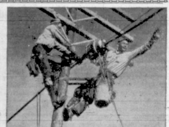
No one can guess the importance of the calls which will flow through the cable these linemen are installing.
