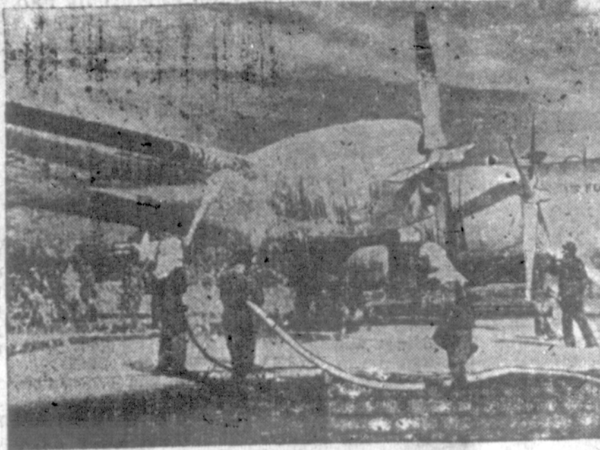
BACK FROM BATTLE . . . Fifth air force crash and fire crews spray the burning engine of a B-29 Superfort with a chemical foam after the medium bomber tangled with enemy jet aircraft and anti-aircraft guns over North Korea. The daring air crew brought the limping Superfort back to this advanced Korean air base without the use of flaps or rudder controls and with two engines out. None of the crew was injured. Our sirmen have noticed an increase in strength of the Reds' air force.
