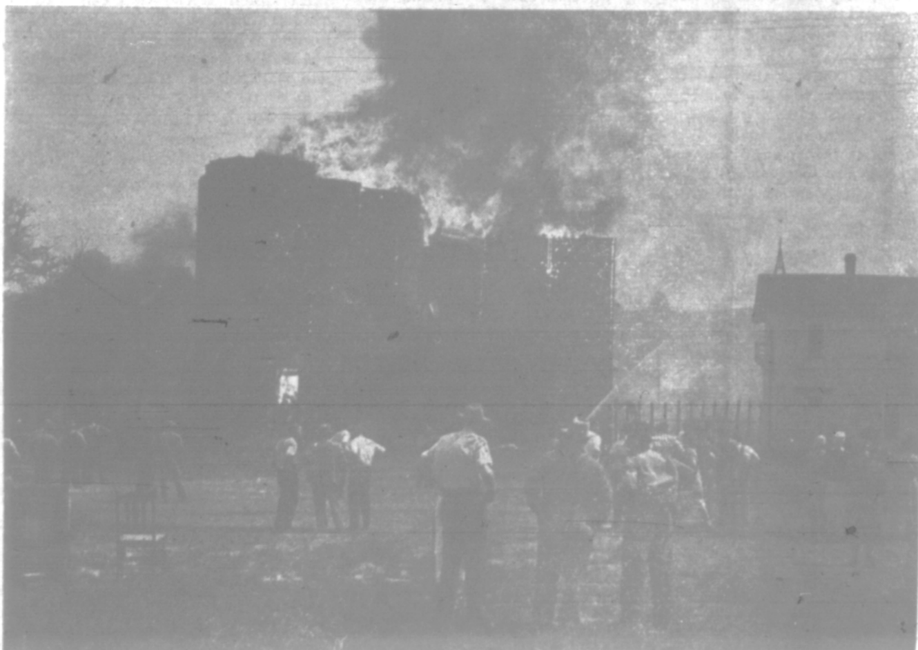
ALL THEY COULD DO WAS WATCH IT BURN. Spectators spent the afternoon watching the flames slowly reduce the elevator to ashes and charred wheat without ability to stop it. Ted Kelley kept the hose playing on the depot while Bill Hall rode the crest with a garden hose, although not in the cut.
