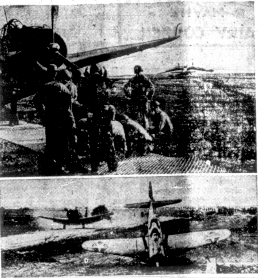
The airport at Safi, French Morocco, offered hard going for navy planes which landed as the field was captured from the French. In picture at top, men are laying a metal strip for takeoff of the torpedo bomber before which they are working. These metal strips have since played an important part in Allied air operations in Tunisia. Below: A navy dive bomber lies nose-down in a ditch near the Safi airport. Another takes off, using the roadway for a runway.
