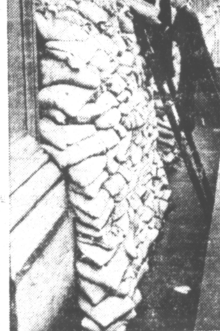
Completing the job of placing sandbags outside the office windows of Hotel Bossert in Brooklyn. The barriers were installed so the hotel organization could keep functioning in case of an air raid.
