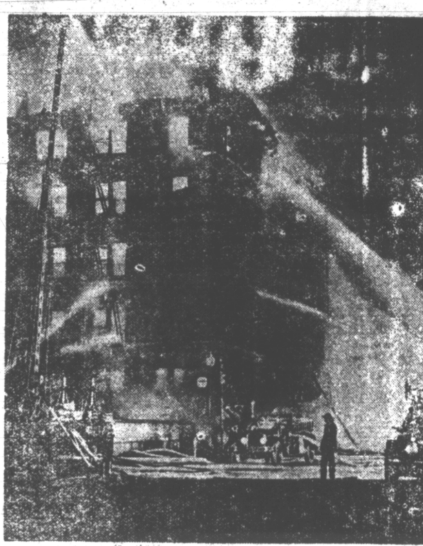
Local fire officials join safety forces throughout the nation in observing National Fire Prevention week, aimed to educate the public for greater care in preventing needless destruction of property by fire. Most fires, like the disastrous one above, could be prevented by constant vigilance against fire hazards. Inspect your home for hazards today, before it's too late.
