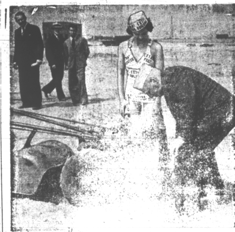
Just an old plowhand was Gov- ernor Frank F. Merriam of Cali- fornia as he broke ground for a $50,000 Press Building at the 1939 Golden Gate International Expo- sition, on Treasure Island in San Francisco Bay. Here he is crank- ing the gasoline plow which he used. Assisting him is Zoe Dell Lantis, Exposition beauty and the "most photographed girl in the world."
