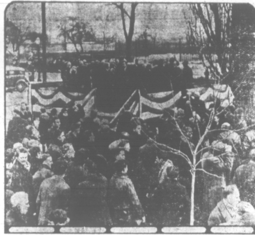
Ground was broken at Euclid, Ohio, a Cleveland suburb, for the nation's first home to be built with funds obtained through the federal home loan plan. Mayor Charles R. Ely of Euclid turned the first shovelful of dirt while several hundred persons looked on. The home will be occupied by F. J. Cook and his family. The photograph shows the crowd gathered for the ground breaking ceremonies.
