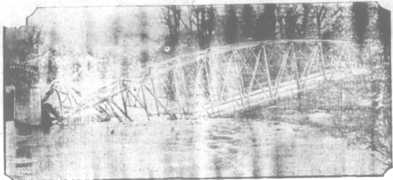
This was a fireproof bridge in the vicinity of Seattle, Wash., but the unexpected happened when a gasoline truck overturned and caught fire. The heat was so great that it melted the steel girders of the bridge, dropping both bridge and truck into the Snoqualmie river.
