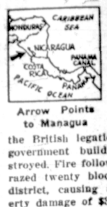
Arrow Points to Managua, American legation, the British legation and Nicaraguan government buildings were all destroyed. Fire following the earthquake razed twenty blocks of the business district, causing an estimated property damage of $30,000,000.
