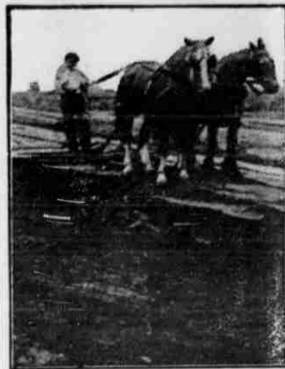
Keeping Road in Good Condition.
