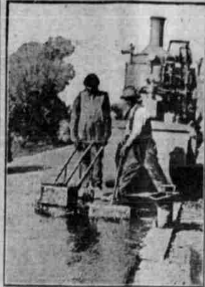
Application of Seal Coat in Progress.
