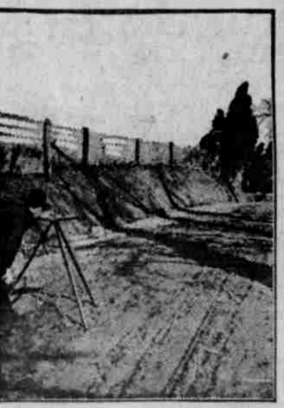
Getting Road Levels Preparatory to Improving Highways.
