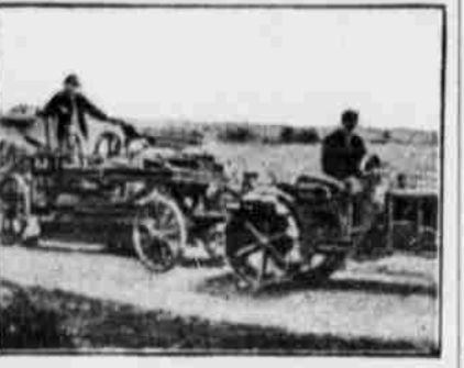
Efficient Aid in Road Repairing.
