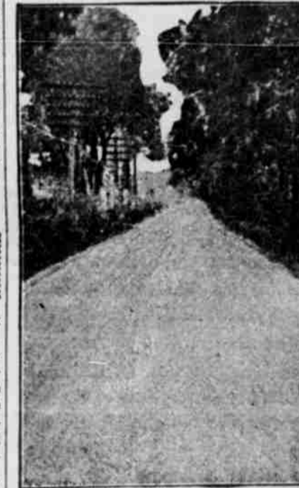
Concrete Road in Mississippi.
