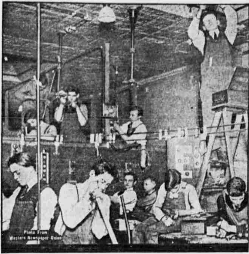
The boys of the United States are doing much to help the country in the war crisis. This picture shows men of tomorrow learning trades at New York's Vocational school. One is doing electric wiring in the shop.
