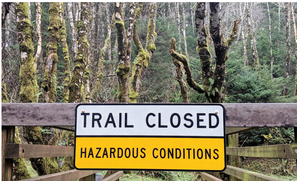
A section of the Oregon Coast Trail in Ecola State Park has been closed after a landslide washed it into the ocean.
