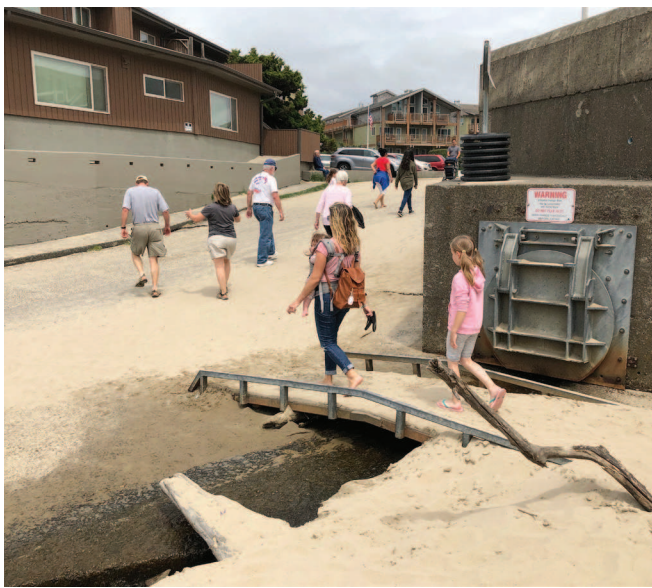
Beachgoers cross a bridge over the Ecola Court outfall in Cannon Beach. Recent samples shows bacteria levels higher than state standards at this location.
