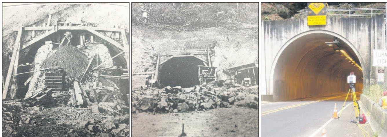
LEFT: Tunnel construction on the south portal, circa 1937. CENTER: Construction at the north portal. RIGHT: Tunnel at a 2010 site visit.
