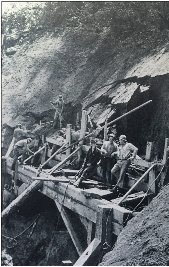
Workers in 1936 at work on the Arch Cape Tunnel.
