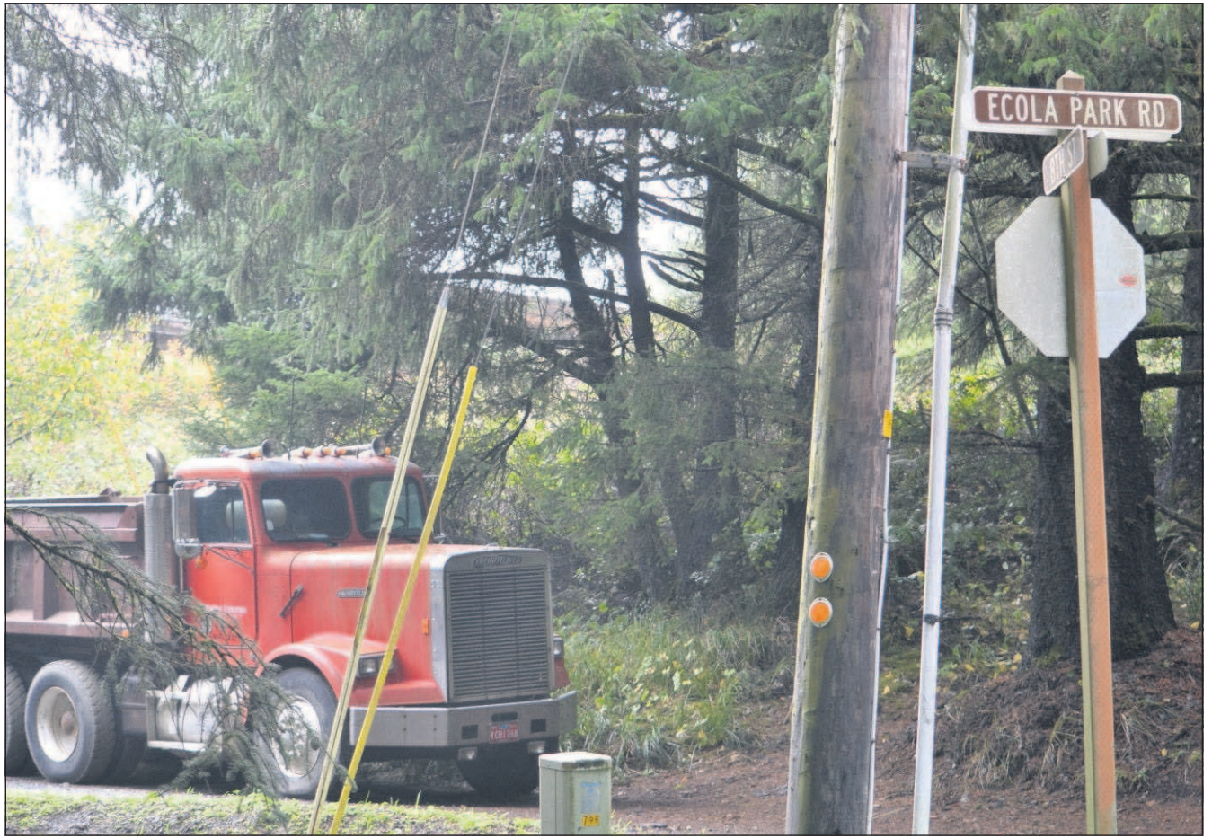
Intersection of Ecola Park Road and 8th Street, where street paving is about to begin.
