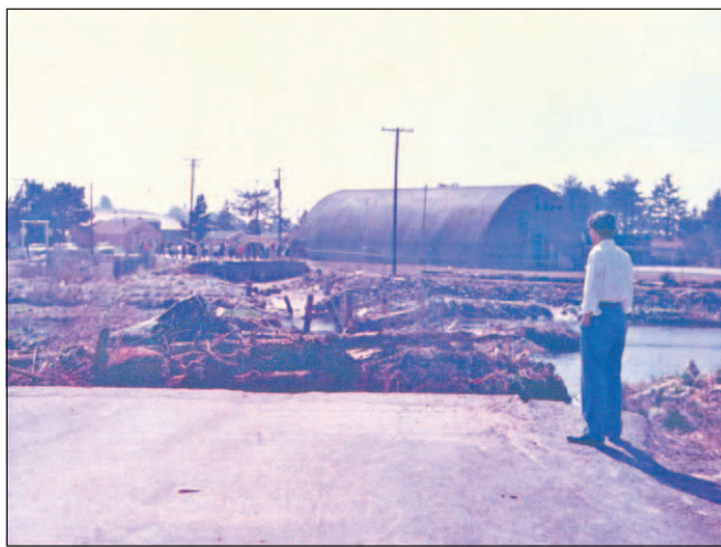
The bridge that crossed Elk Creek on the north side of Cannon Beach collapsed during the 1964 tsunami. The school's gym is visible on the south side of the creek, as well as students from Cannon Beach Elementary School lined up to look at what remained of the bridge's footings.
