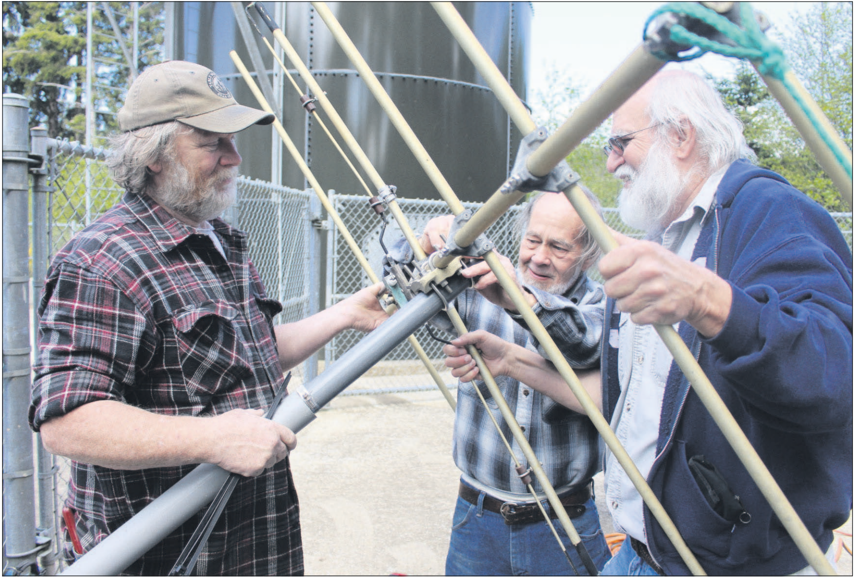
From left: Roger Bassett, Gordon Spalding and Ray Merritt make adjustments to an antenna before connecting it to the KMUN translator (not pictured). The translator had been relocated from a private garage on Elk Mountain Road to the north-end to test the signal.
