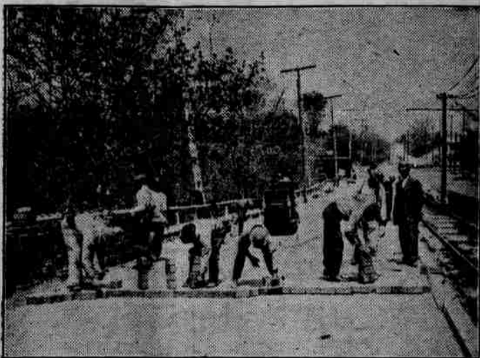
Laying Vitrified Brick for Country Road Pavement.
