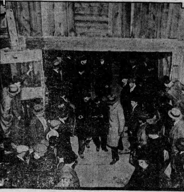
Eleven were killed and more than fifty injured in a fire which swept a sanitary district sewage tunnel in Chicago, trapping the unfortunates 35 feet underground.
