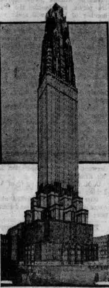
Architects' drawing of the proposed Fashion building to be erected on or near Fifth avenue in New York city. It will be of polished terra cotta blocks of various colors and will be the first skyscraper in full color.
