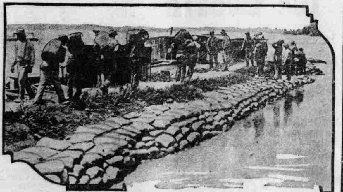
The railroad transfer of Vicksburg was in great danger of destruction by the flood waters of the Mississippi and an army of men was put to work reinforcing the levee with thousands of sacks of dirt.
