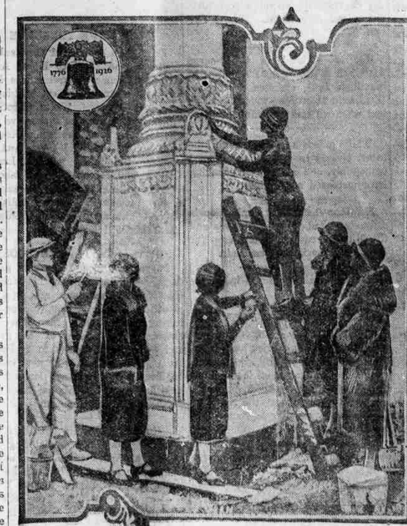
Young women artists turn from their jars of color and paint brushes to assist plasterers in setting ornaments in place atop huge pylons which adorn the main entrances to the Palace of Agriculture and Food Products, of the vast exhibition buildings which forms a part of the great Sesqui-Centennial International Exposition being staged in Philadelphia from June 1 to December 1 to celebrate the 150th anniversary of the signing of the Declaration of Independence. Climbing ladders and walking along rickety scaffolds is nothing new to these young ladies, but each time they do it they get a thrill.
