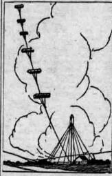
string of kites to an altitude of 1,600 feet. Messages transmitted from the set of field wireless attached to this kite-supported aerial were received 150 miles away with distinctness, al-though the ordinary range of the set was only 25 miles. One thing that aided materially in obtaining this resuit was the fact that the kites flex so steadily that the aerial was always maintained at a constant altitude.
