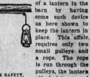
pulleys, the lantern FOR SAFETY. attached to one end and then pulled up to a convenient height, the loose end of the rope being fastened to a cleat on the wall. If this device is arranged in about the center of the barn much better light will be given than if the lantern were carried around from place
