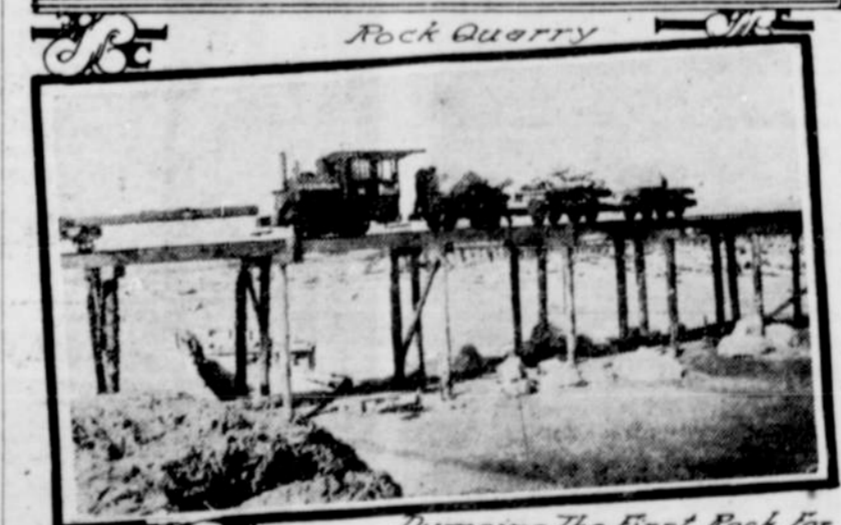
Dumping The First Rock For Jetty
