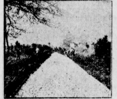
MACADAM ROAD CONSTRUCTION. (From Southern Good Roads, Lexington, N. C.)
